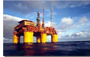
Energy (Oil & Gas)
